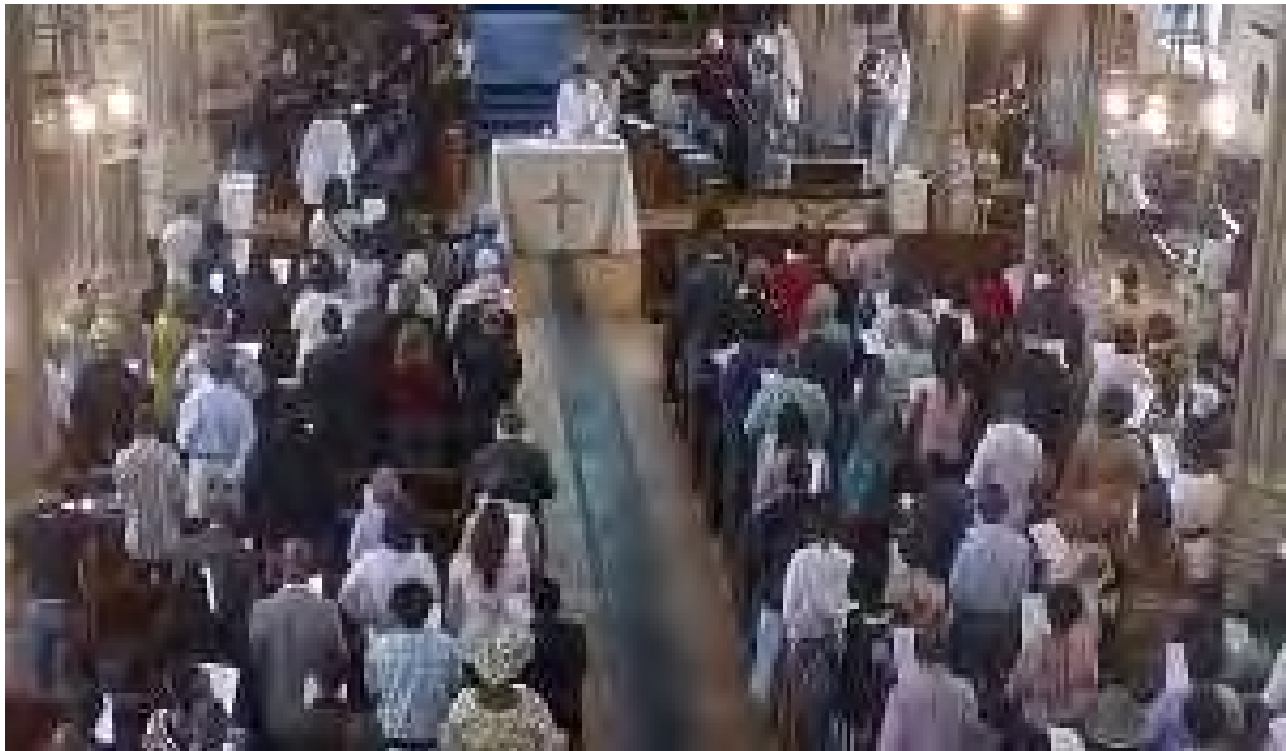
A bird's eye view of the Sunday morning Service on 6 th July 2008, taken from the scaffolding erected to allow repairs to the West Wall of St. John's. (Photo by Adrian Clarke)
